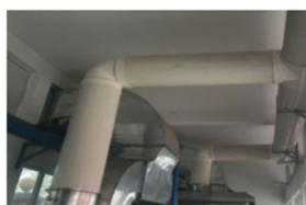
**Waste heat insulation pipe**
