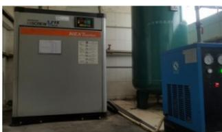
**Variable frequency rotary screw compressor**
