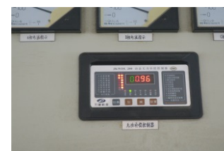
Power factor auto-compensation device
